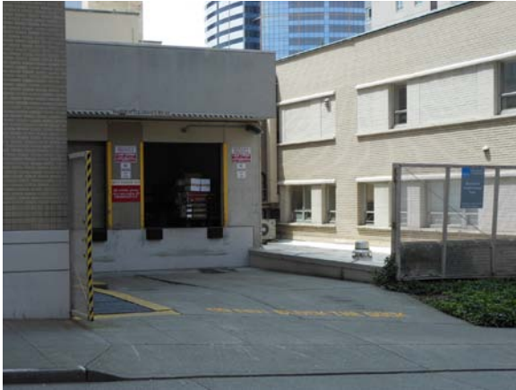
Design service areas so that they can be screened from the street.
