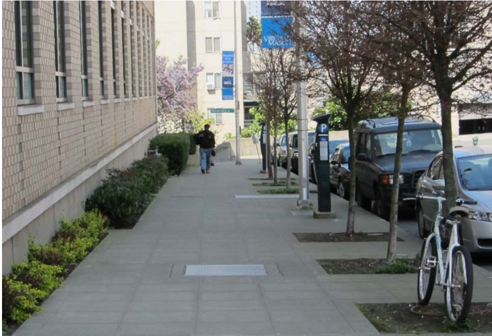
View of Ninth Avenue, looking north - existing condition.
