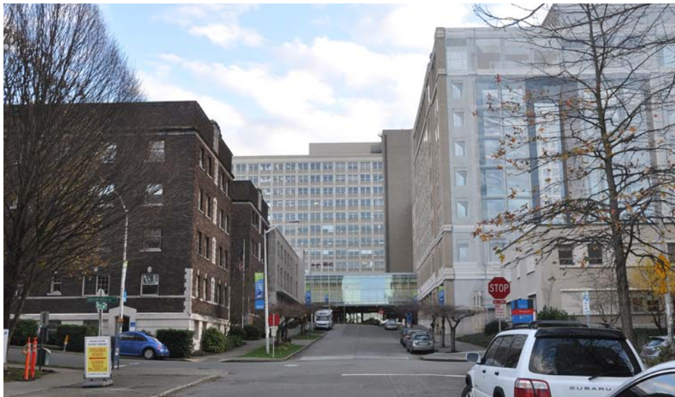
View of Terry Avenue, looking south - existing condition.
