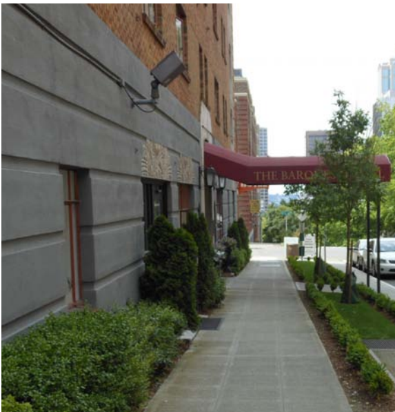
Retain the sense of scale and welcome along the block between Terry and Boren.
